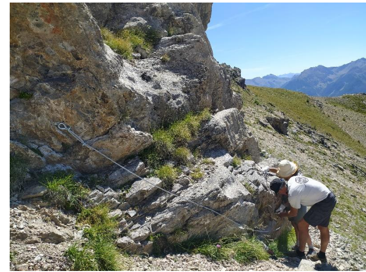
Installation main courante ©A.Merdrignac
