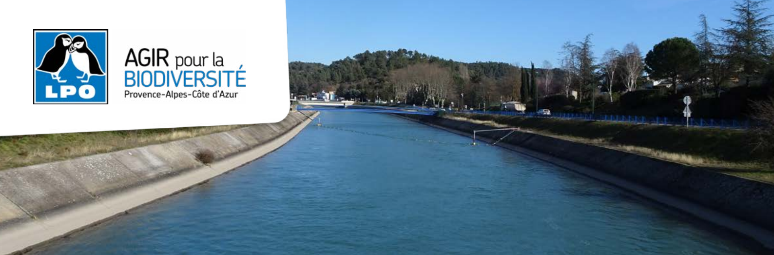
Canal EDF © LPO PACA
