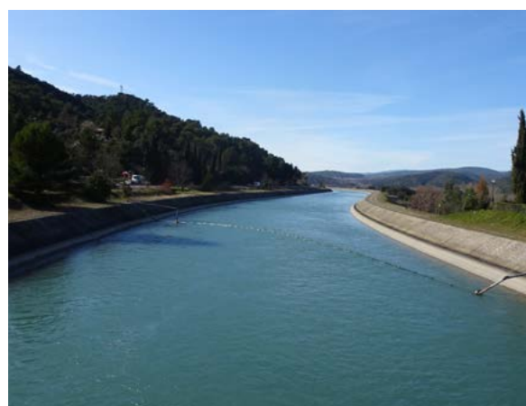
Canal EDF © LPO PACA
