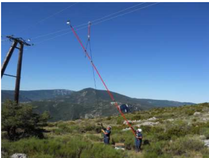
“Firefly” beacons and installation on a subtransmission line in Rougon (ERDF)
